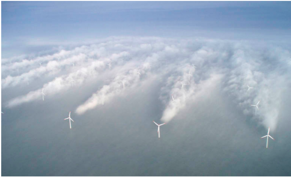
Photograph showing the “ wake effect ” at the Horns Rev off-shore wind farm off the shores of Denmark. Source: Hasager et al. (2013)
